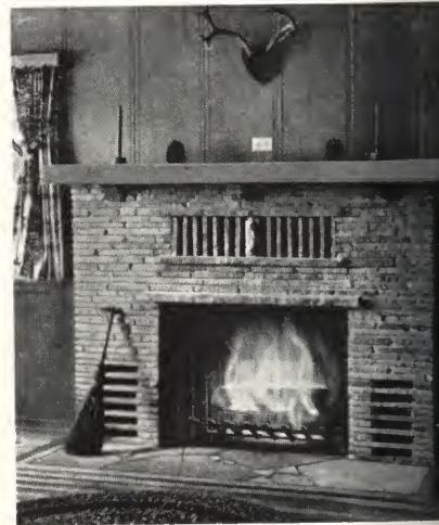
7. Cool Air Intakes and Warm Air Outlets. Front Built of Split Stone.
